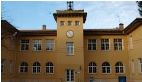
Telemedicine Research Unit
